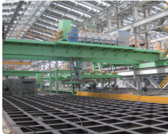
SERVICE WELDING MACHINE
