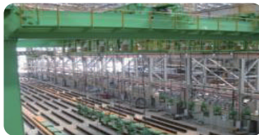
5 WELDING SERVICE GANTRY
