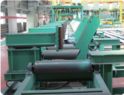
2 IN FEEDING CONVEYOR
