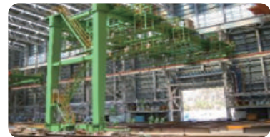
6 WELDING SERVICE GANTRY
